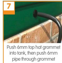
Push 6mm top hat grommet into tank, then push 6mm pipe through grommet
